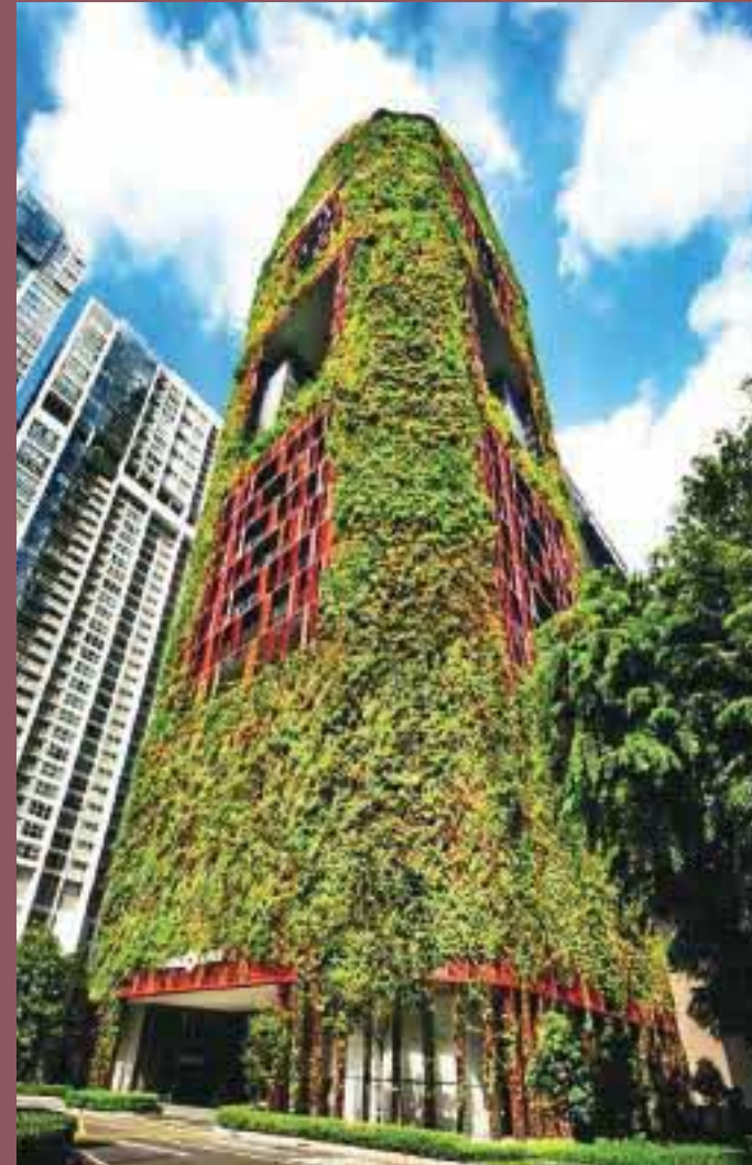
The Oasia Hotel Downtown features sky terraces and cascading lush planting integrated into the building form, providing green visual relief for guests and employees.
